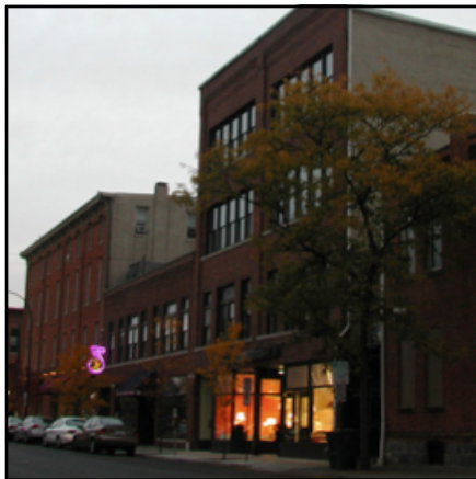
Schwaben Hall Renovation Ann Arbor, Michigan
