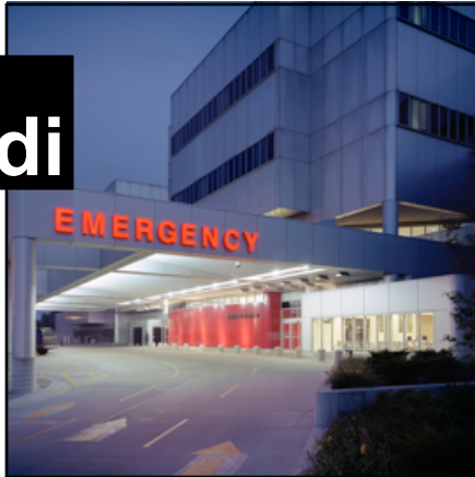
Detroit Receiving Canopy
