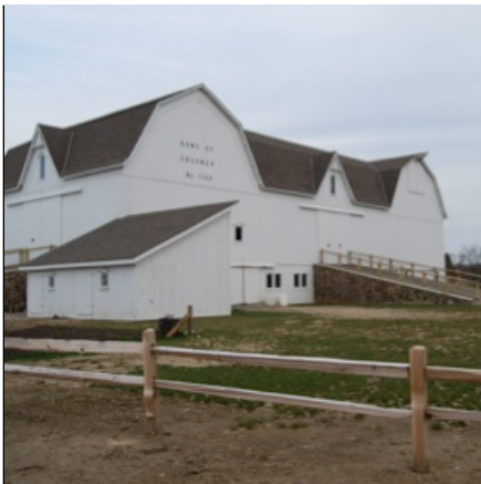
Ellis Barn Re-Located
